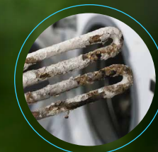
buildup clogs appliances & water heaters
