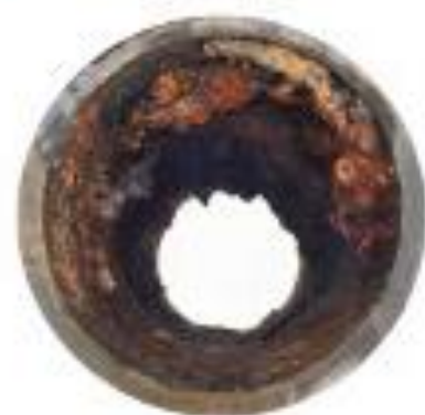
Reno underground water pipe
